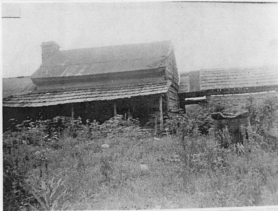
Log house on "river road" near Farmers, Ky. Once occupied by John Cassity Family and married daughter Rosa Cassity Elam. House was razed during the building of Cave Run Lake.
